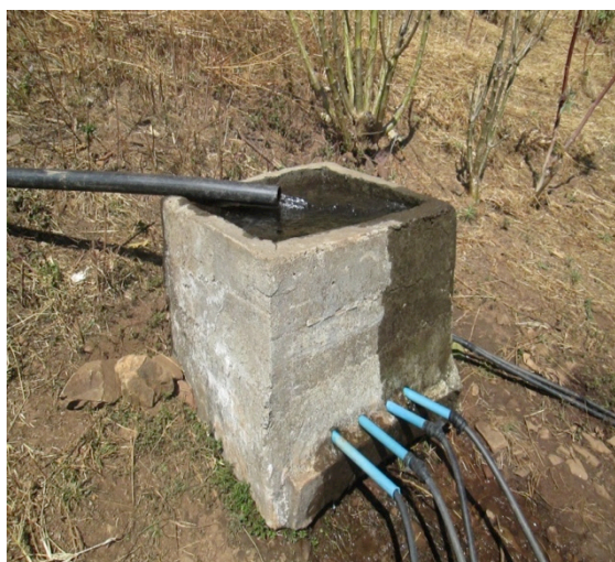
Photographs 12 and 13 - Typical village collection tanks, distribution system and multi-purpose water points
