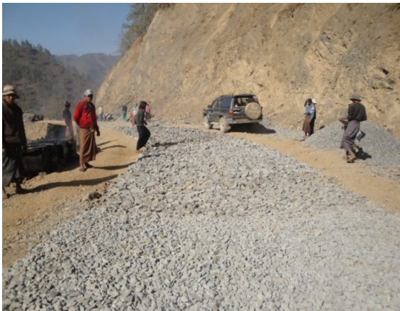
Sub-base/base course laying
