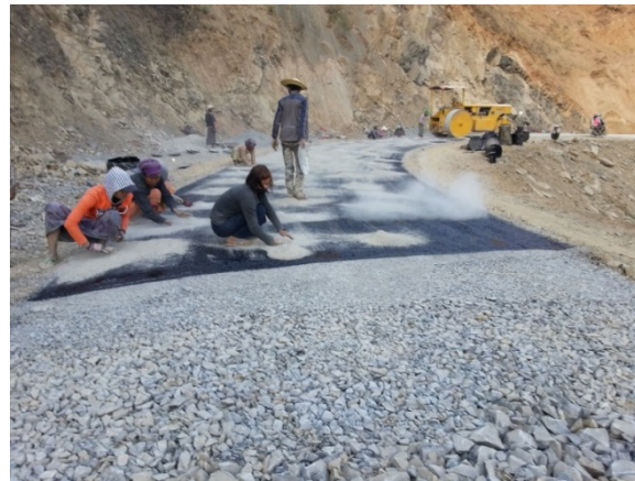
Laying of seal coating
