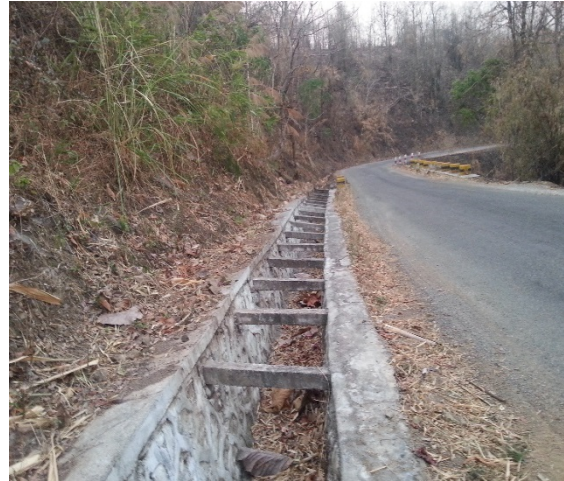
Paved road with proper water management (Kyaukhtu-Mindat Road)
